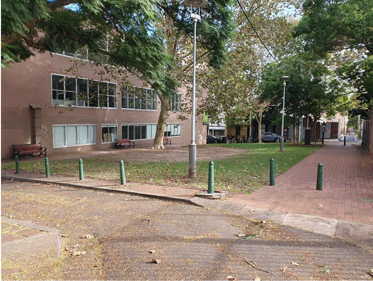
Lower Cooper – Looking north to Cooper Street. The turf is heavily worn out under the canopy of both the existing mature trees. Paths are in a good condition with some tree root lifted paving around the Plane tree. One bollard is dislodged. Existing benches are in good condition. Lighting is at end of life.
