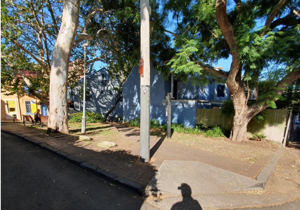
Adelaide Street Reserve – looking southwest towards Adelaide Street from Little Riley Street. Turf is in poor condition due to pedestrian traffic and shade from mature existing trees. Paths are in a good condition with some tree root lifted paving around Eucalyptus tree. End of life lighting and signage is visible.
